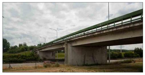
The cross-section of the bridge must remain the same as the current cross-section, with a total width of approximately 10 metres. The length of the bridge is approximately 90 metres, in three spans. The new design may possibly use four spans by placing an additional pillar in the central reservation.
