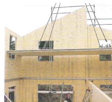
Ceiling assembly with floor-to-roof exterior walls
