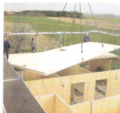
Ceiling assembly in floor-to-floor exterior walls
