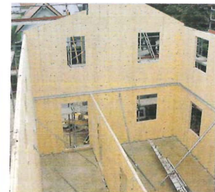
View of the superstructure without the ceiling
