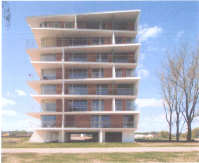
3 floor has been reserved for parking. ↓ The deep overhangs double as solar shading.
