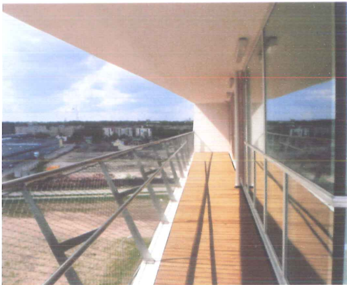
3 floor has been reserved for parking. ↓ The deep overhangs double as solar shading.
