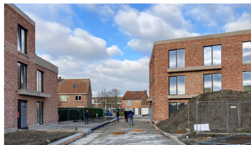
Huisvestingsproject in Bredene, i.s.m. Tech3.
