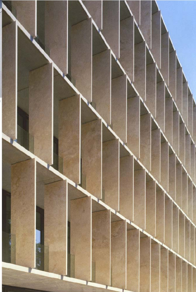
ETH E-SCIENCE LAB ZÜRICH, BAUMSCHLAGER - EBERLE
