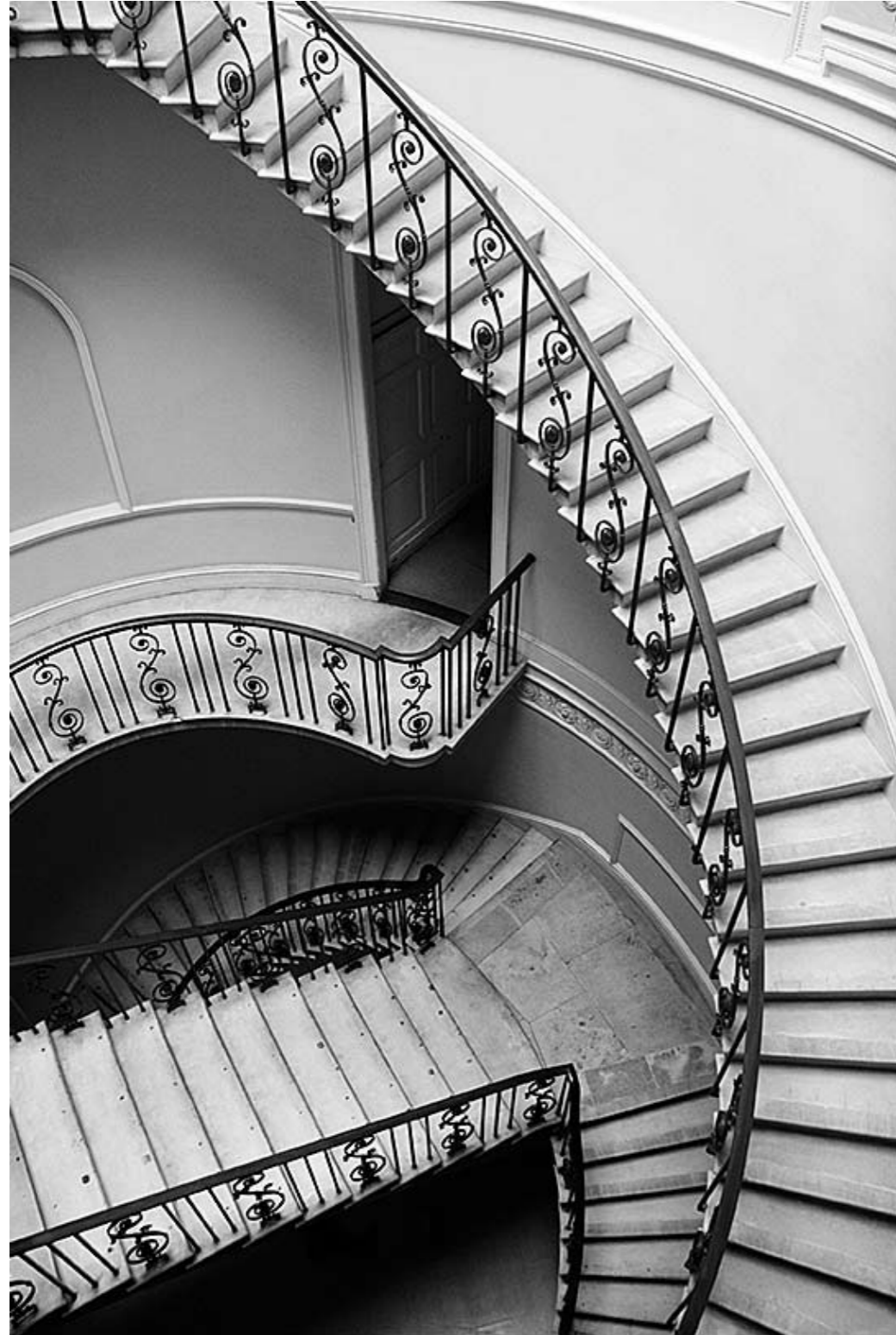
Nelson stair, Somerset house , Londen
