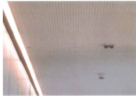
perforated plasterboard / acoustic active
