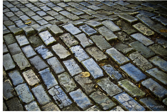
Fig 10. Buitenverharding Scoria bricks
