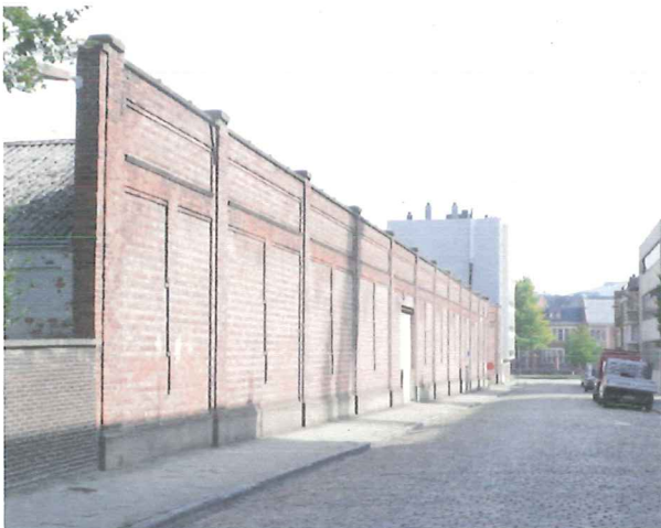
Site photograph of the old textile factory wall along Nonnemeersstraat.
