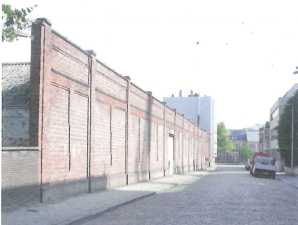
Site photograph of the old textile factory wall along Nonnemeersstraat.
